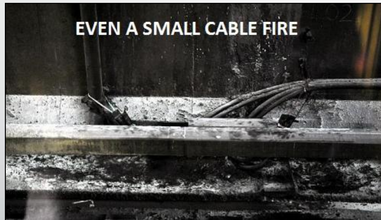
Singapore MRT 2013 - Newton Underground Station. Cable overloaded and caught fire
