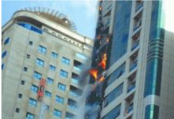
A fire gutted 17 floors of a 33-storey residential building in the Al Nahda area of Sharjah
