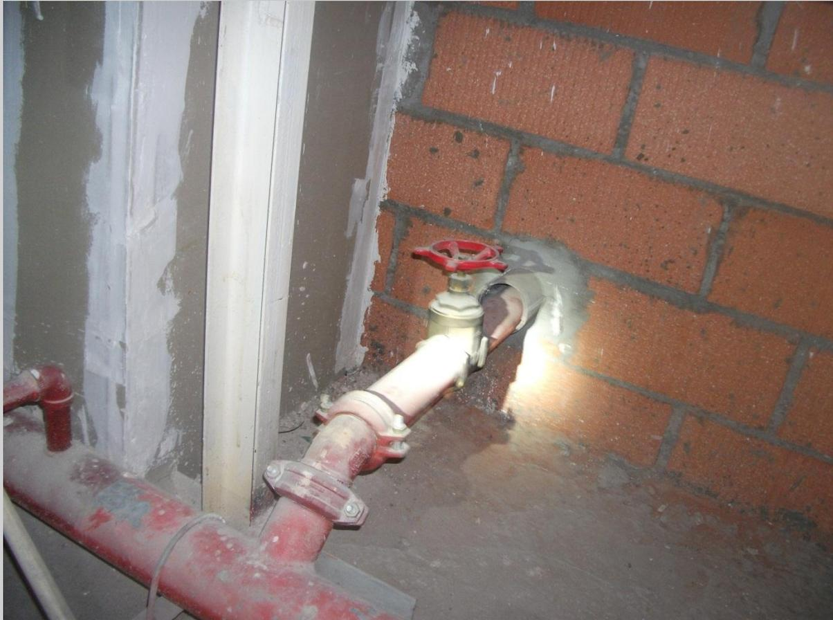
Tenant Isolation Valve for sprinkler system outside tenant boundary line in the Mall's mechanical space.
