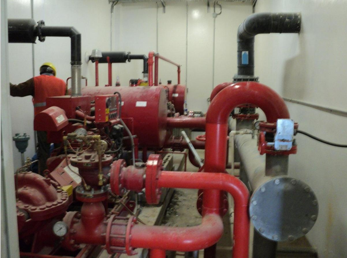
How will the fire pump be Replaced, Removed or Serviced when you have to climb into the room?
