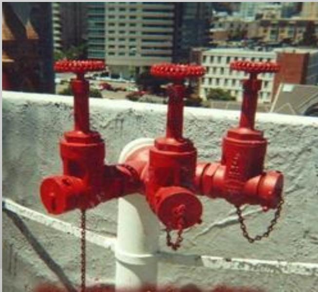
Roof Manifold for Class I
