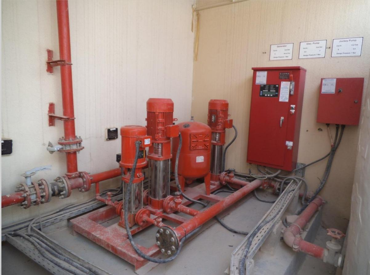
How will the fire pumps be Tested with no gauges, no means to measure RPM, and no test header?
