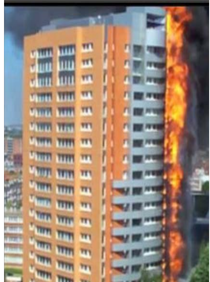
Mermoz Tower – France (2012)
