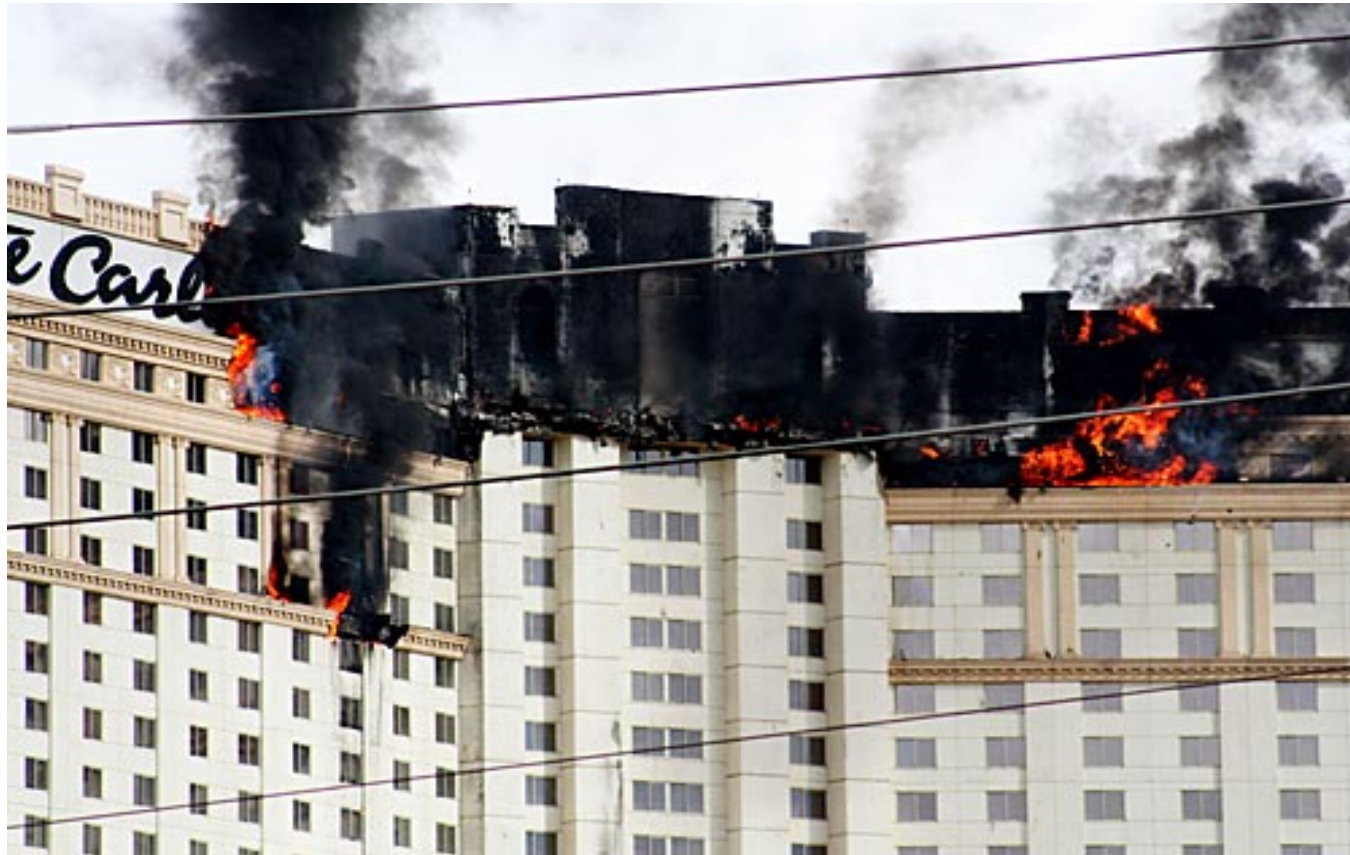
Monte Carlo Casino Fire – Las Vegas January 2008 Damage – est. $100 million
