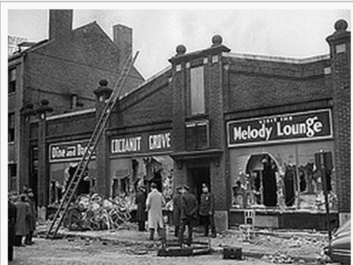
The front of the Cocoanut Grove nightclub after the fire
