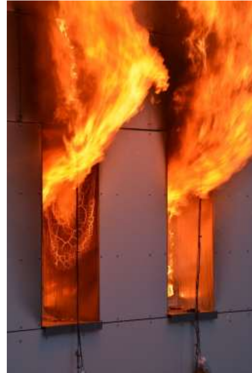
Flashover fire for Facades...
