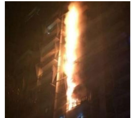
Lacrosse tower fire, Melbourne
