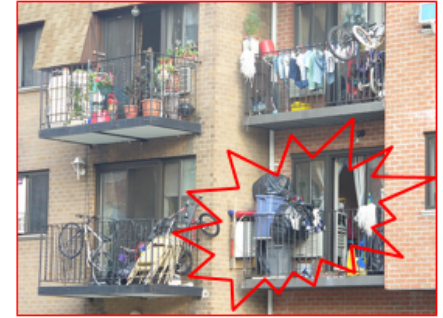
Façade Ignition Sources
