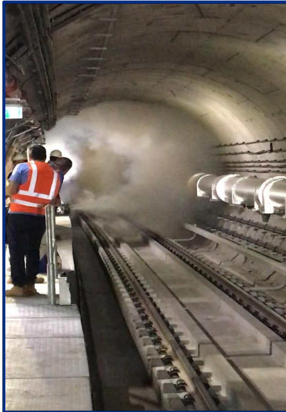
Tunnel – Smoke Test
