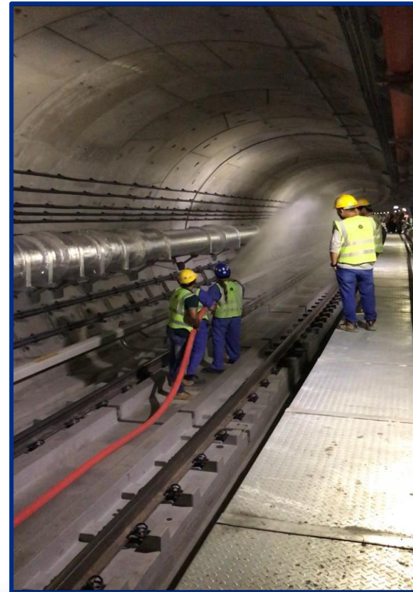
Tunnel – Landing Valve Test
