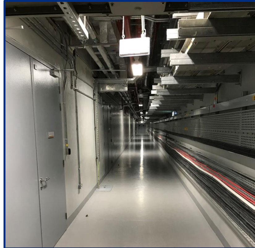
Service – Basement Level 3
